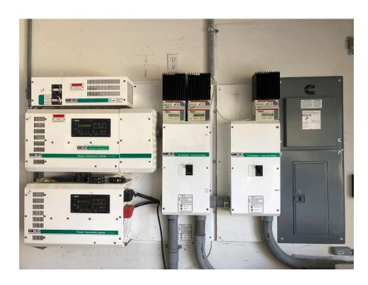
Most of my house runs on the inverters continuously. You will notice in the picture there is a 100 amp transfer switch that transfers the Oven, Washing machine and a few other items to the inverters on a power outage. Note 2 trace inverters 4 KW each in a 240 configuration.
