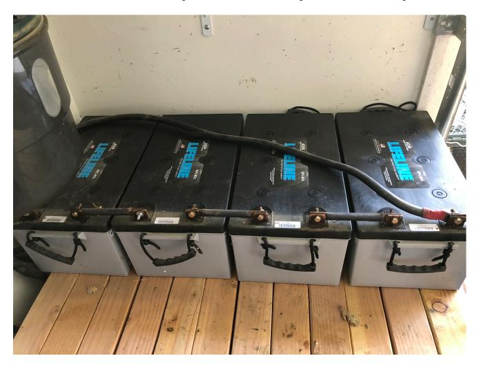
Note that most battery connections between batteries are insulated copper tubing. If you look on-line, it will give you the amperage rating of copper tubing. This will run my house and radio equipment for a long long time on both 120 & 240 volts
